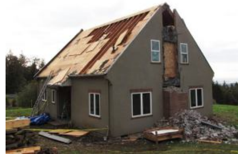
Seventy percent of the construction waste from the outdated and drafty English-style cottage was diverted from landfills.
